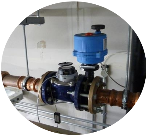
Water meter and valve assembly installed at the incoming water mains.
